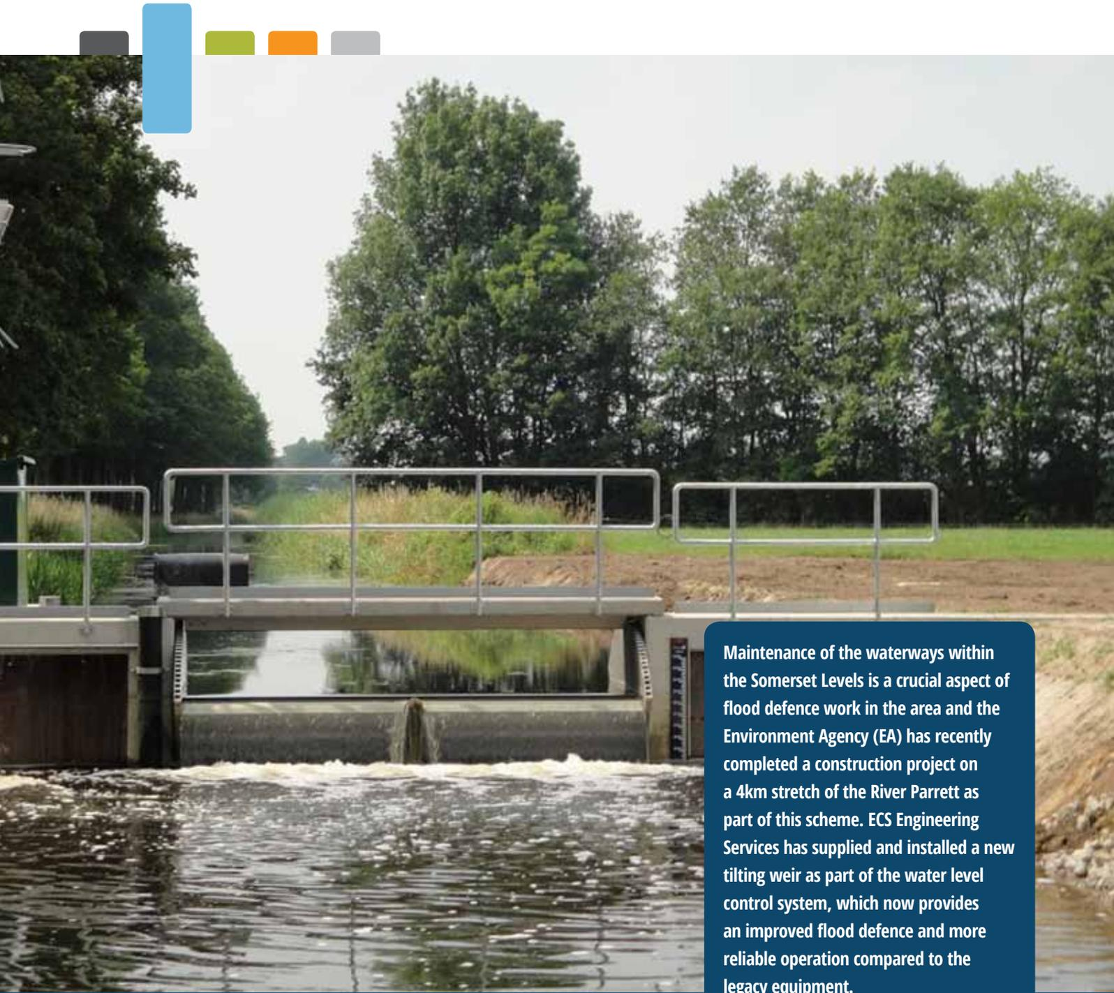
**Maintenance of the waterways within the Somerset Levels is a crucial aspect of flood defence work in the area and the Environment Agency (EA) has recently completed a construction project on a 4km stretch of the River Parrett as part of this scheme. ECS Engineering Services has supplied and installed a new tilting weir as part of the water level control system, which now provides an improved flood defence and more reliable operation compared to the legacy equipment.**
