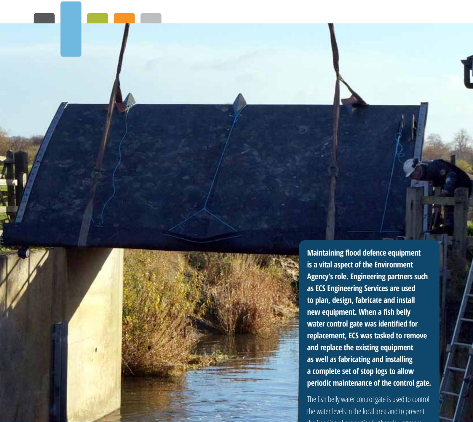
**Maintaining flood defence equipment is a vital aspect of the Environment Agency's role. Engineering partners such as ECS Engineering Services are used to plan, design, fabricate and install new equipment. When a fish belly water control gate was identified for replacement, ECS was tasked to remove and replace the existing equipment as well as fabricating and installing a complete set of stop logs to allow periodic maintenance of the control gate.**
