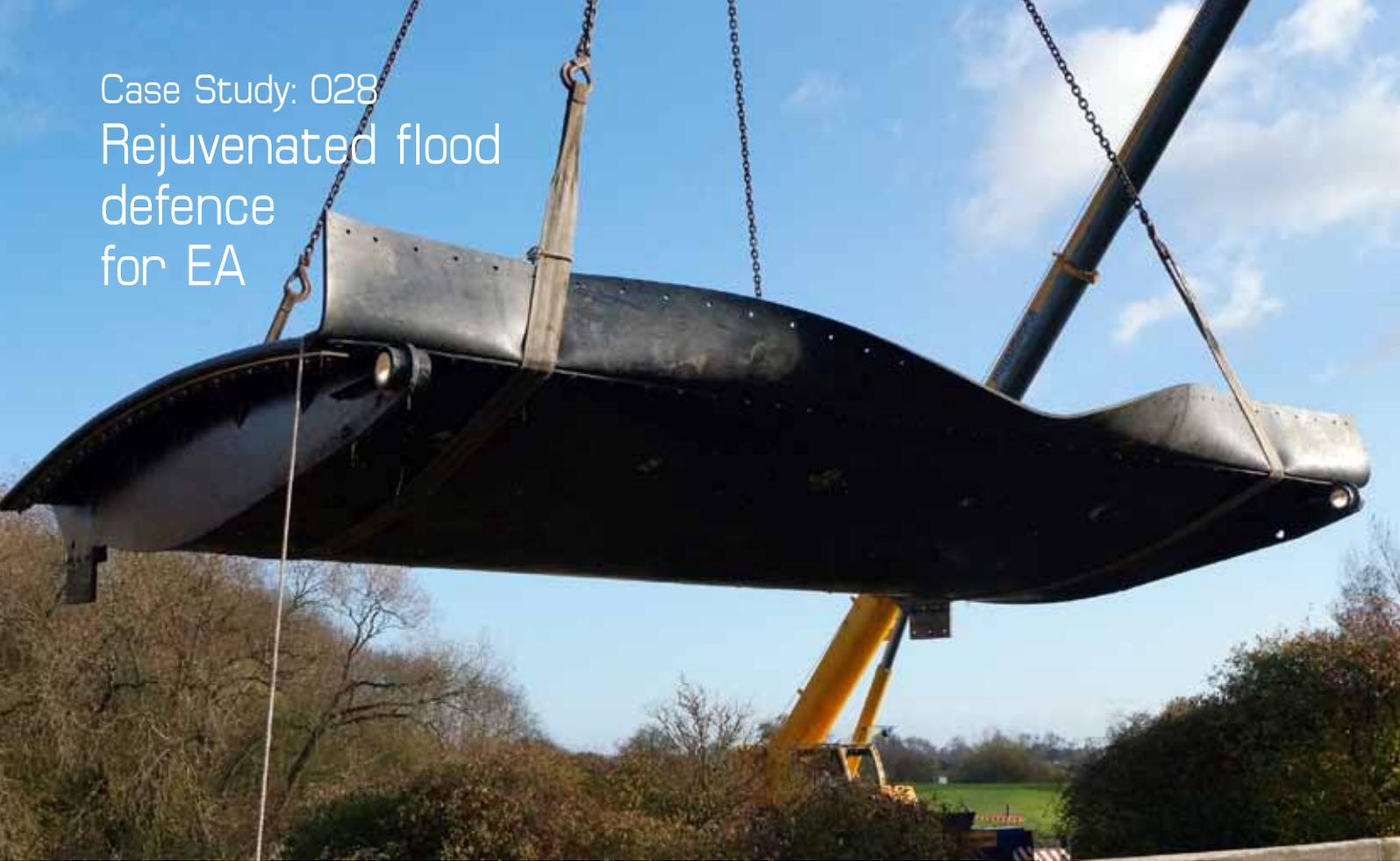
The project was scheduled to be completed during the summer months when the water flow through the control gate was at a minimum and therefore the risk of flooding at its lowest. The first steps involved careful measurement of the existing control gate and drawing up the designs for both the replacement control gate and the stop logs before the fabrication department could start on manufacturing the new components.
