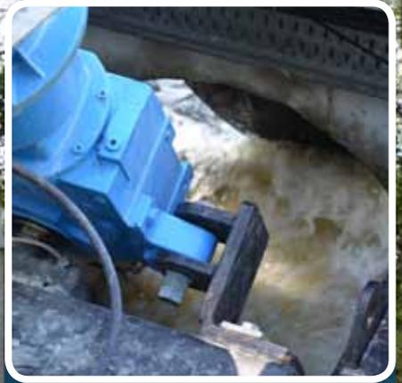
The motor and gearbox combination is matched specifically to this application and is driven via a variable speed drive to provide optimum efficiency
