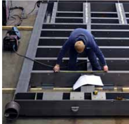
Framework in construction
