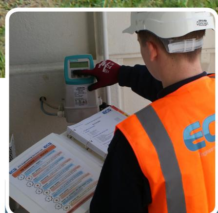
The latest water level and flow measurement devices were installed to ensure reliable operation of each pumping station
