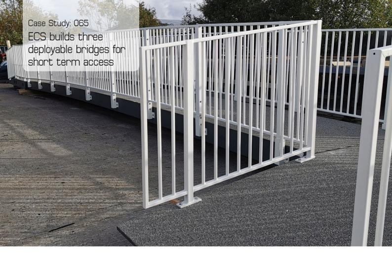
Other than length they are all essentially identical, being 1.8m wide between the parapets and designed for foot, bicycle and wheelchair users. Each has a factory-applied silica anti-slip coating resin bonded to the deck and complies with the safety and robustness requirements of Eurocode 0 (EN1990 para 2.1 & 2.2) concerning impact, damage resistance and quality control.
