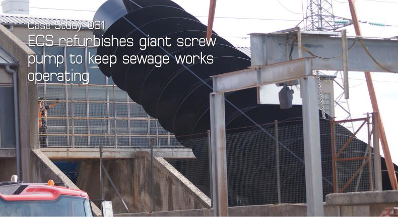
An inspection showed that the drive gear was still good condition, but the screw body was heavily worn, so ECS developed a plan that retained the motor and the gearbox while the time-expired parts were replaced.
