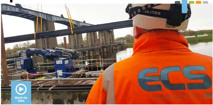
ECS Engineering Services has been continuing its renovation of Colwick Sluice in Nottinghamshire for the Environment Agency, by repainting the aging upstream steelwork at the site. The business has blasted and repainted I-beams and hand railings at the sluice on the River Trent, ensuring that the site is adequately protected from corrosion.
