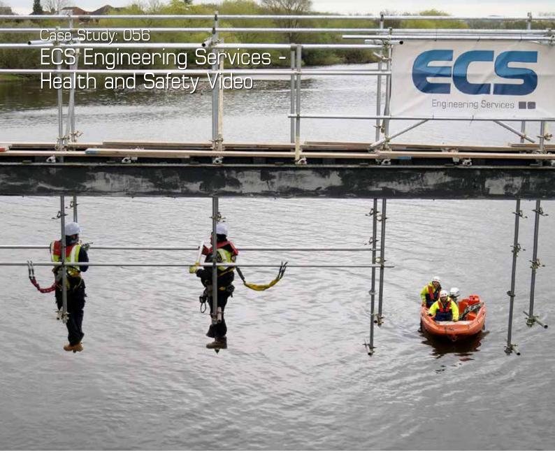
In order to do that we work safely and securely. The Environment Agency's current, pro-active maintenance and renewal programme for river structures and water management infrastructure - has brought us to Colwick Sluice, where: in order to refurbish the 'steel' structure of the large sluice gate system in the river Trent, there is a requirement to deploy additional river safety measures — during the assembly and disassembly of the scaffold system.
