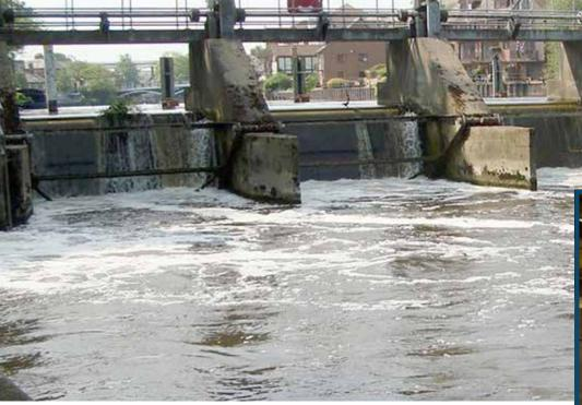
ECS was contracted to produce one 2.38m wide x 1.13m high and eight 2.68m wide x 4.43m high radial gates for installation by their inhouse engineers at the weir. The entire design process of each gate was carried out inhouse by ECS, with all designs adhering to BS EN 1090-2 certification. The gates were required to geometrically match the existing gates at the weir and mirror their crest level, preserving the water dynamics through the weir.
