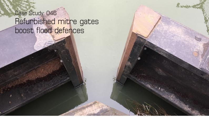
The existing wooden mitre gates were showing signs of wear after many years of service, so to carry out refurbishment work, they needed to be removed and transported to the ECS fabrications centre in Nottinghamshire. However, accessing the gates was a considerable challenge, as the central sluice required dewatering and damming before work could begin in earnest.
