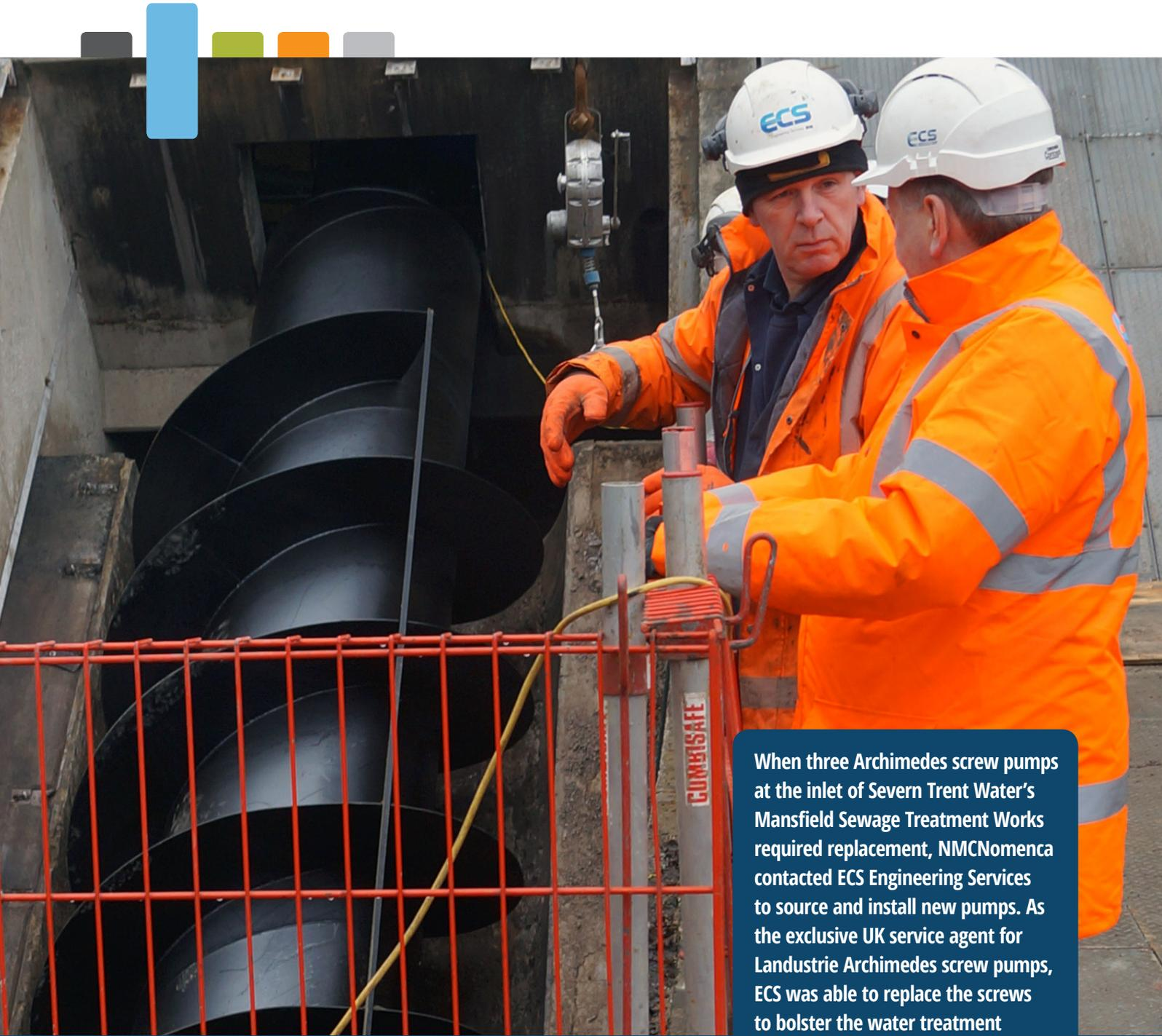
When three Archimedes screw pumps at the inlet of Severn Trent Water's Mansfield Sewage Treatment Works required replacement, NMCNomenca contacted ECS Engineering Services to source and install new pumps. As the exclusive UK service agent for Landustrie Archimedes screw pumps, ECS was able to replace the screws to bolster the water treatment infrastructure at the site.
