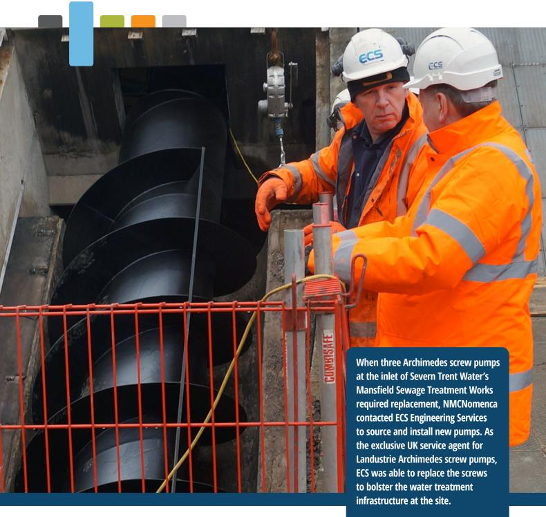
Archimedes Screw Pumps boost local water infrastructure Mansfield Sewage Treatment Works lies adjacent to the River Maun, processing the majority of effluent water from farms and homes in the surrounding area. The three original screw pumps at the inlet station had been operational since the 1970s, and were displaying a drop in efficiency due to overall wear.
