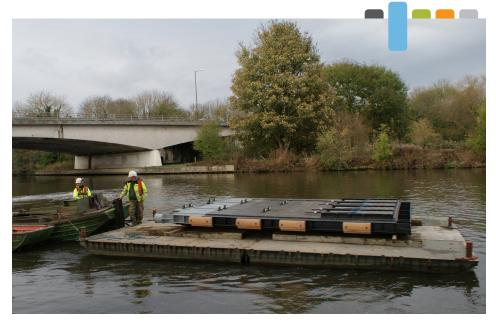
As part of a £1.8 million investment in the refurbishment of a number of its assets along the River Thames, the Environment Agency (EA) has replaced the lock gates at both Romney and Marlow. This complex part of the project was delivered by ECS Engineering Services as a turnkey solution that involved considerable in-house design and steel fabrication work.
