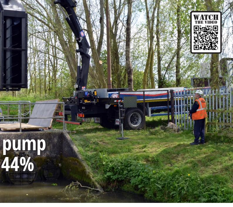
Initial calculations suggested that the new screw pump should deliver an energy saving of 40%. However, Natural Resources Wales wanted confirmation of this and so the actual energy savings were closely monitored over a 6 month period and compared to the submersible pumping syste. The Archimedes screw pump is in fact delivering a 44% energy saving.
