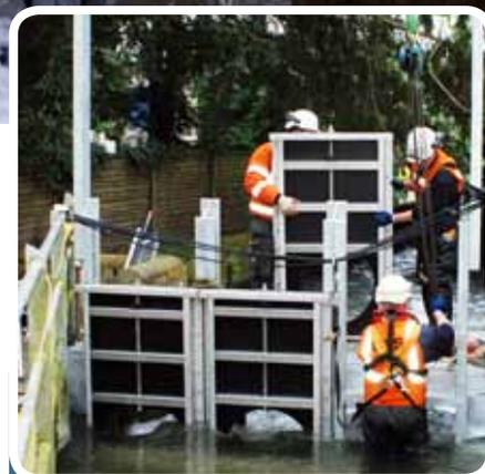
**The main framework of the new sluice is built from galvanised steel, while the penstocks are made from High Density Polyethylene (HDPE)**
