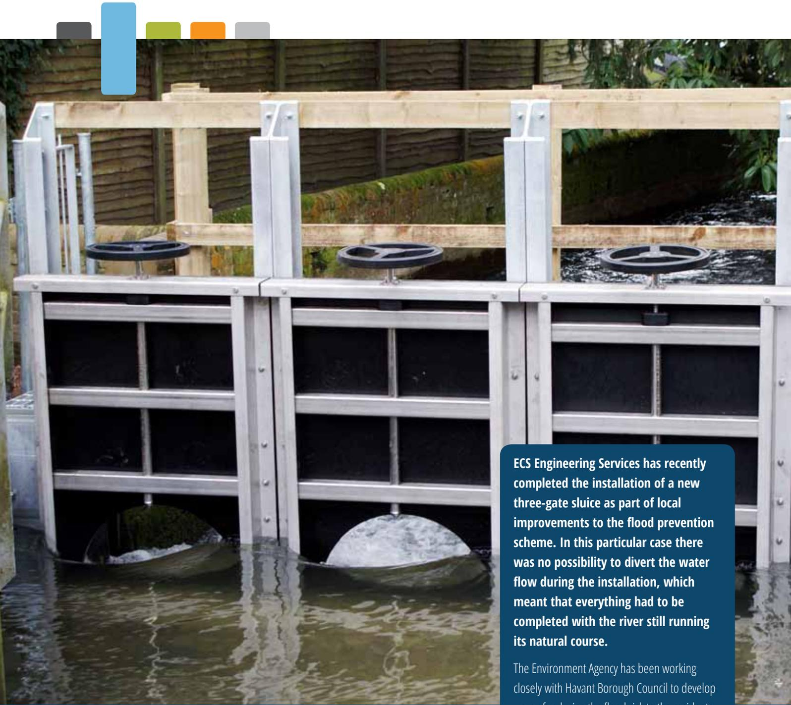
**ECS Engineering Services has recently completed the installation of a new three-gate sluice as part of local improvements to the flood prevention scheme. In this particular case there was no possibility to divert the water flow during the installation, which meant that everything had to be completed with the river still running its natural course.**
