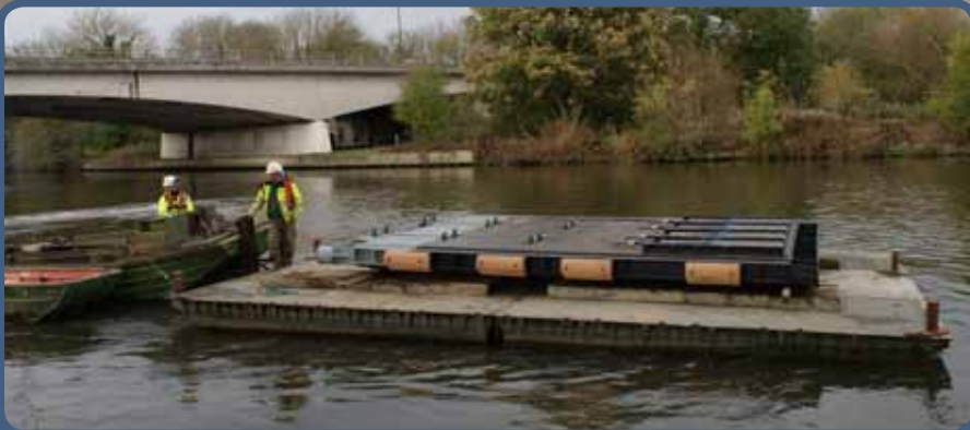
Under BS EN 1090, both sets of lock gates will be CE certified and installed by the experienced ECS engineers.
