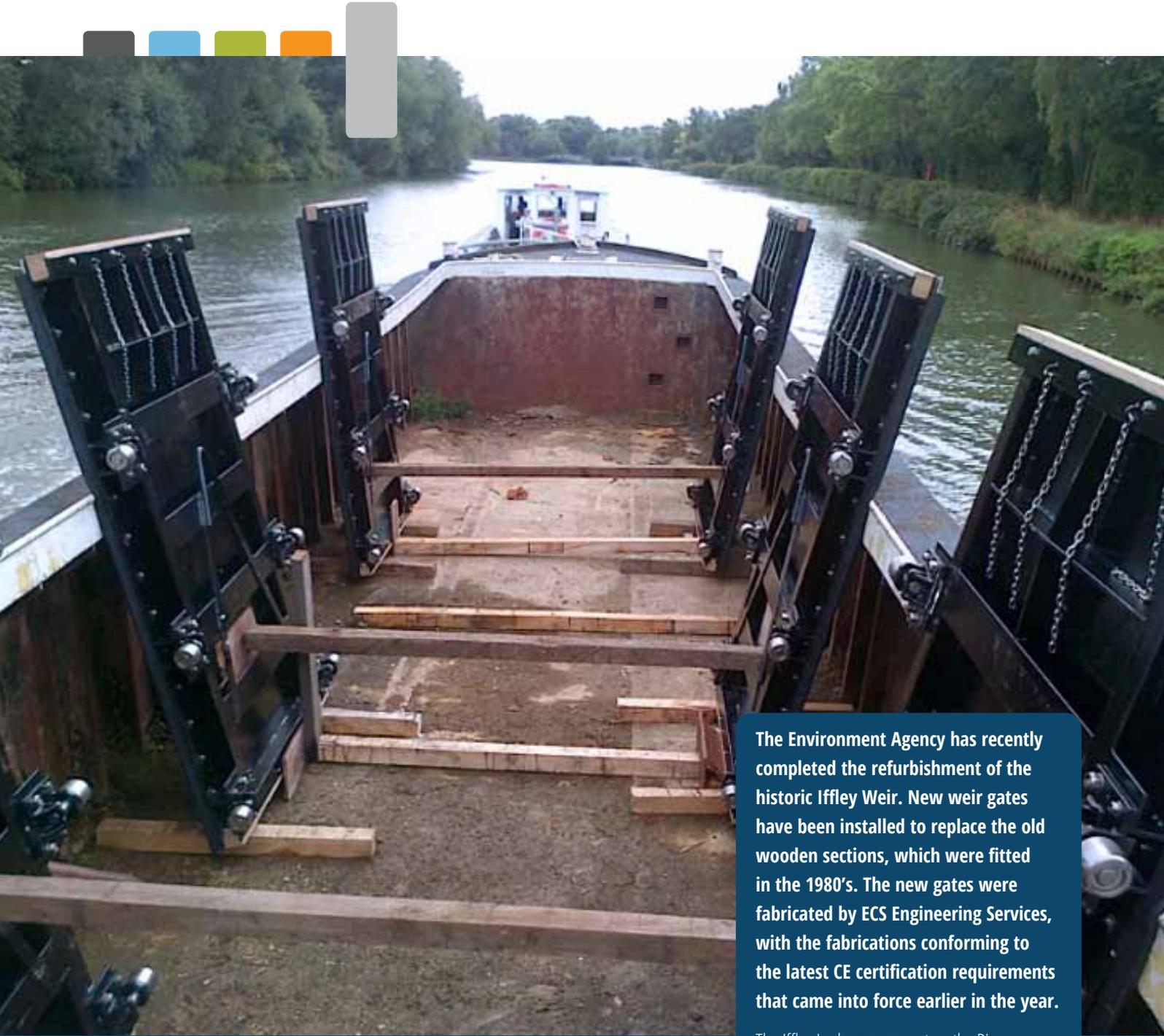
**The Environment Agency has recently completed the refurbishment of the historic Iffley Weir. New weir gates have been installed to replace the old wooden sections, which were fitted in the 1980's. The new gates were fabricated by ECS Engineering Services, with the fabrications conforming to the latest CE certification requirements that came into force earlier in the year.**
