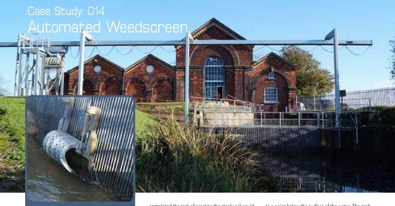
The EA brought in ECS Engineering Services to deliver an improved, more reliable solution which would reduce maintenance costs and provide an automated weedscreen solution.
