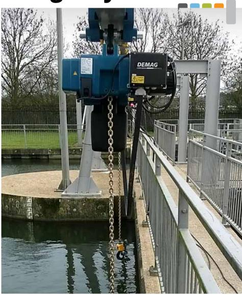
Improving the design height of the lifting beams also had a knock-on effect on the electrical system, as well as the control building itself. Given the weight of the stoplogs and the hoists, the designers had to ensure that there was no vibration or deflection in the vertical plane when the system is in use.
