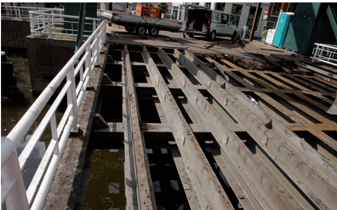
Deck refurbishment: the original timber deck has caused the supporting steel structure to be in bad condition.
