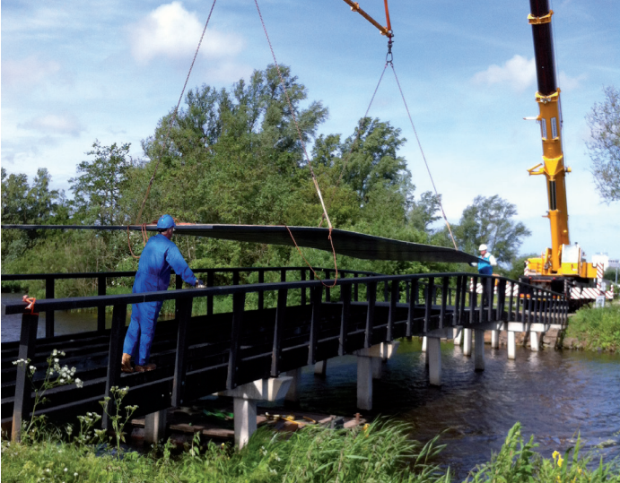
Installation of a 15x4m InfraCore® Inside deck.
