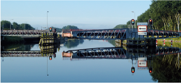
This heritage swing-bridge in Souburg was refurbished and fitted with InfraCore® Inside decks.
