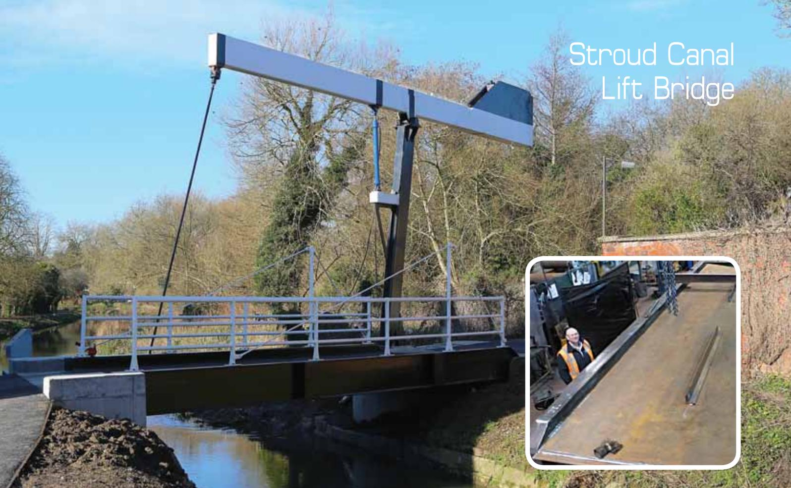
Replacing a road bridge over a water course is already a complex task, and in this case there were additional factors such as a restricted work space and narrow access routes that would have to be used by the large plant equipment required for the project. In addition, the road approaches the canal at an angle and this had to be considered in the final design.
