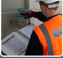
The latest water level and flow measurement devices were installed to ensure reliable operation of each pumping station
