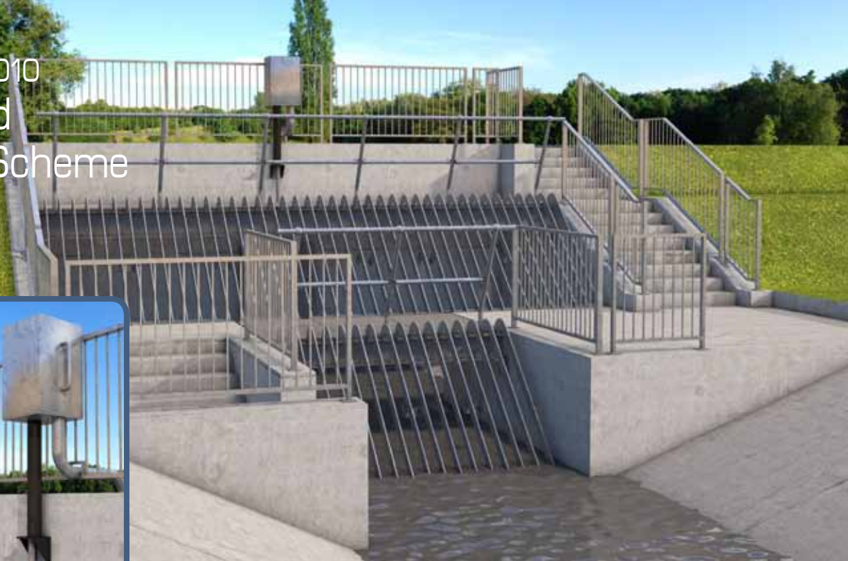
A hydraulic actuator is powered by pressurised oil and provides a 4-20mA position signal back to the control panel
