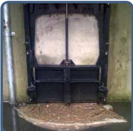
The actuator will be used to control the new cast iron penstock, which was supplied by Waterfront Fluid Controls
