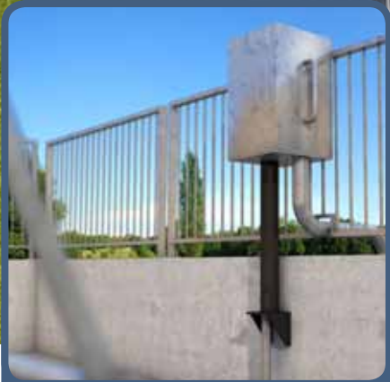
A hydraulic actuator is powered by pressurised oil and provides a 4-20mA position signal back to the control panel
